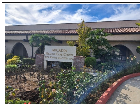
arcadia care center入口處
