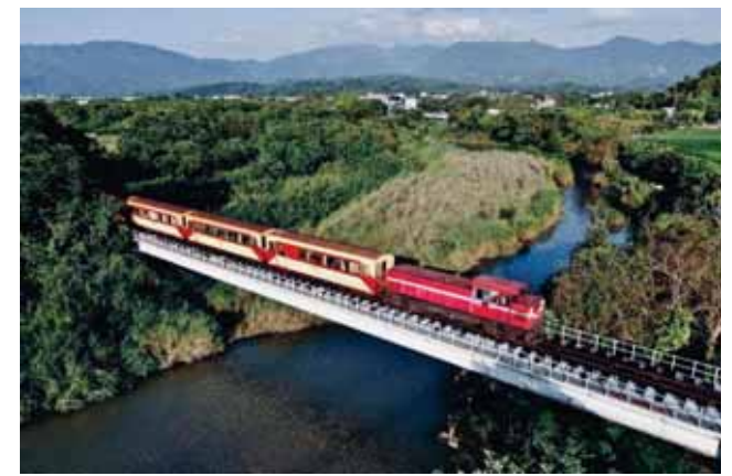
Alishan train running across the bridge
