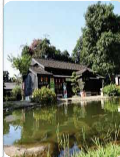
Dormitory for sawmill workers
