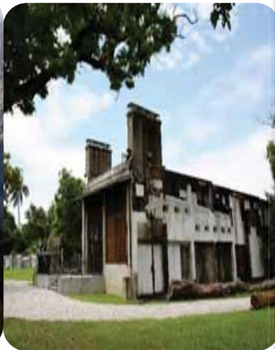
Sawmill for timber processing
