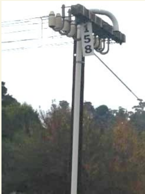
Telephone Pole 158 = PBM158 PBM207
