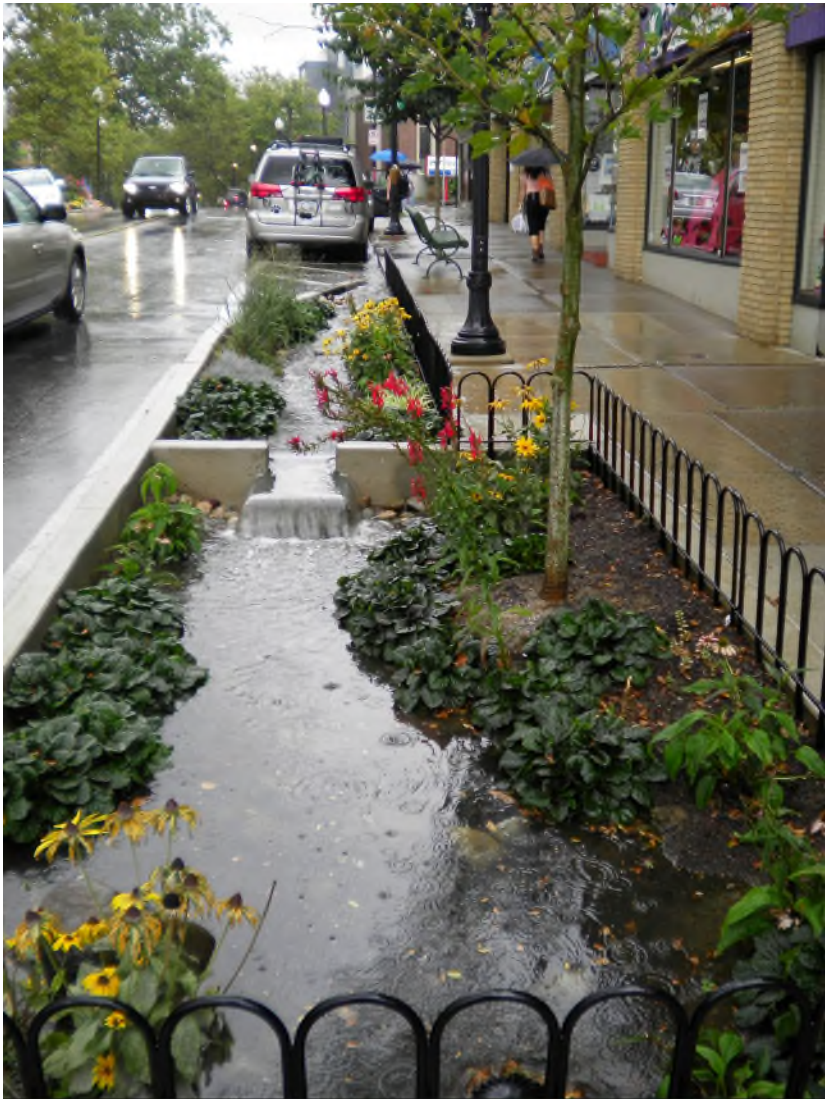
Typical rain gardens/bio-retentions
