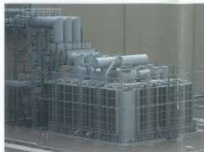
■ 電子炉用変圧器 1000VA 220/200V 3φ 50Hz Transformer for nuclear power station
