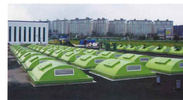
Cheonan STP (South Korea) Capacity : 70000m 3 /d Operation : 2008~ Application : Municipal
