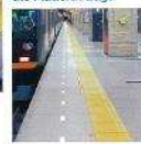
Flash Light Strip along the Platform Edge
