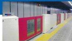
Partial-Height Platform Screen Doors
