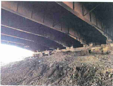
Abutment north half
