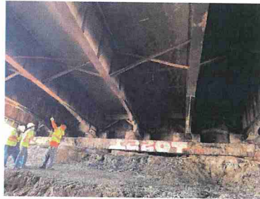
Abutment south half
