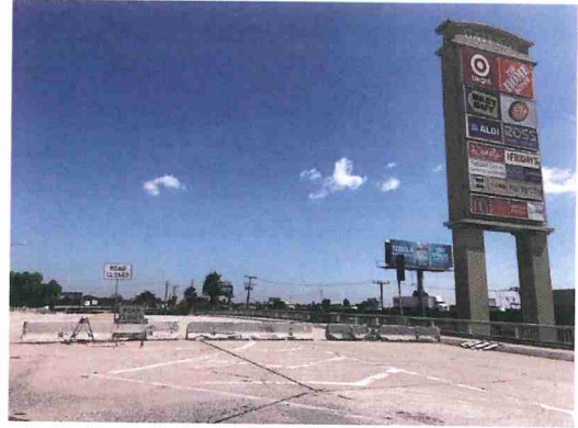
P2_K-Rail was moved back to original position _ Done
