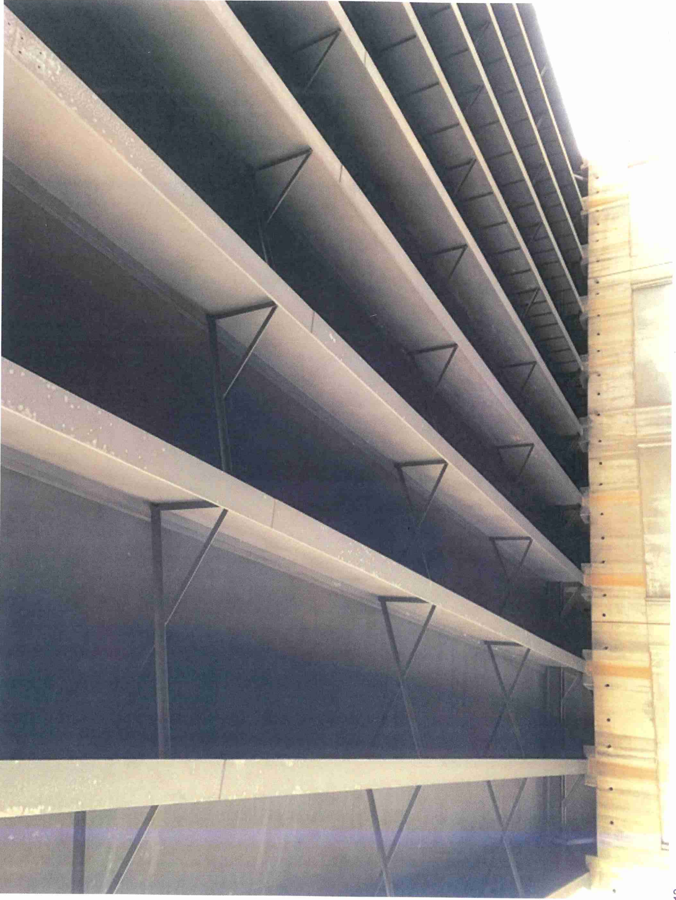
Photo #12 Underside Photo
