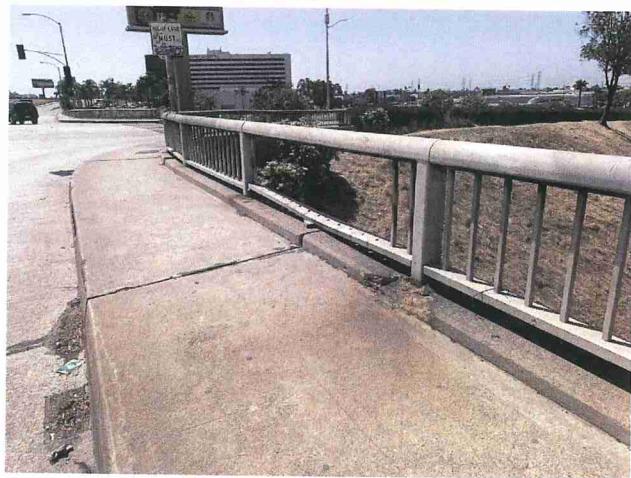
Photo 8 Missing Balusters
