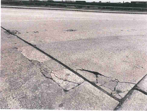
Photo 4 Joint Spalls
