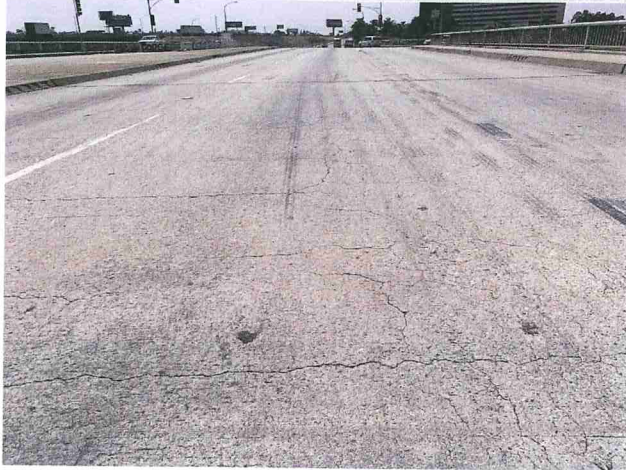
Photo 3 Deck Cracking
