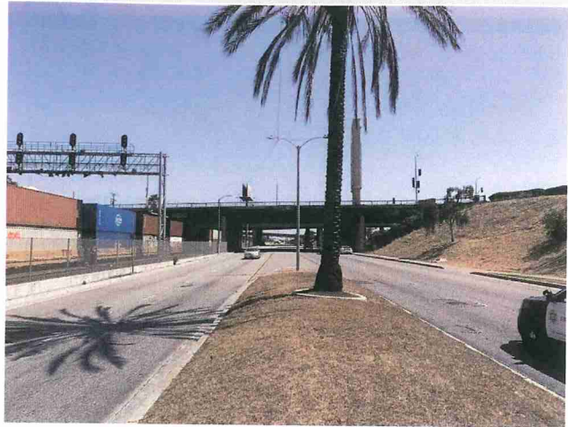
Photo 10 Elevation View from North
