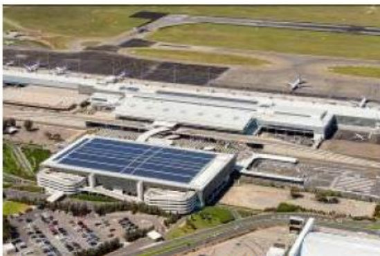
Figure 1: Adelaide Airport 1.17MW Solar Installation
