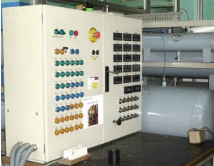
Components Repairs: Pneumatic Equipment
