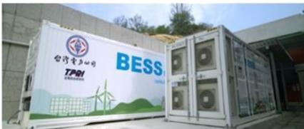
Fig.3 The 2MW/1MWh short duration application EESS II
