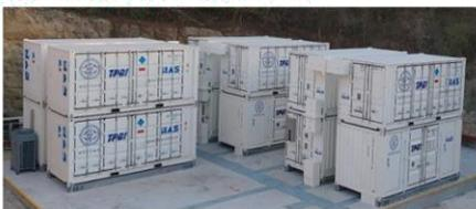
Fig.1 The 1.8MW/10.8MWh long duration application EESS I
