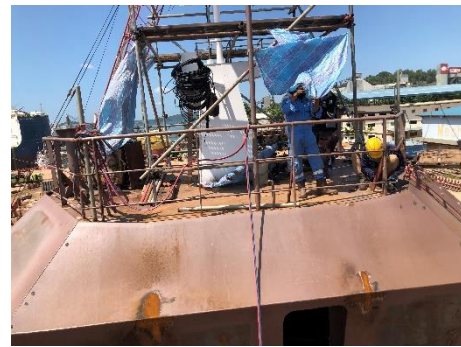
桅桿電纜線安裝
