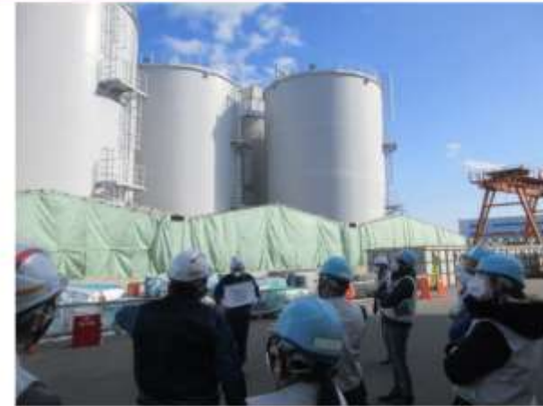
K4 tank area
