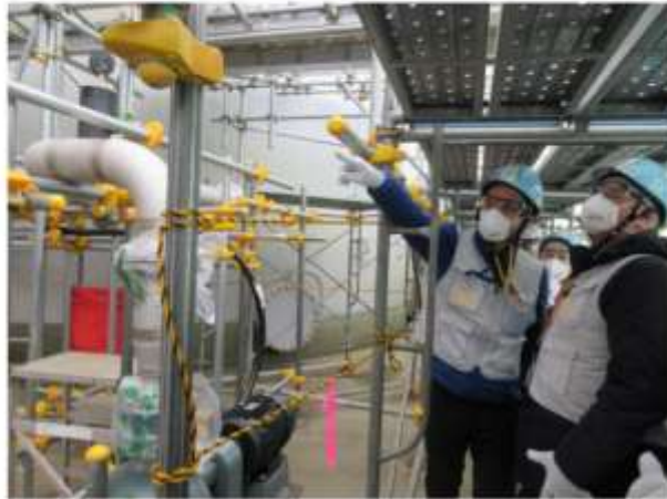
K4 tank area
