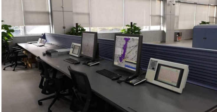
I4D Control Position In Guangzhou Control Center
