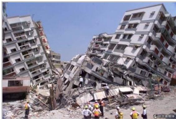
51,711 Houses Destroyed 53,768 Houses Damages
