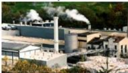
Industrial power stations
