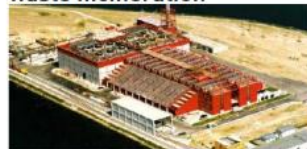
Thermal waste treatment plants, waste incineration
