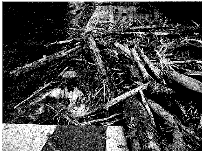
Examples of catching driftwood by open-type check dam
