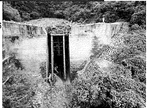
No.2 dam (After debris flow)
