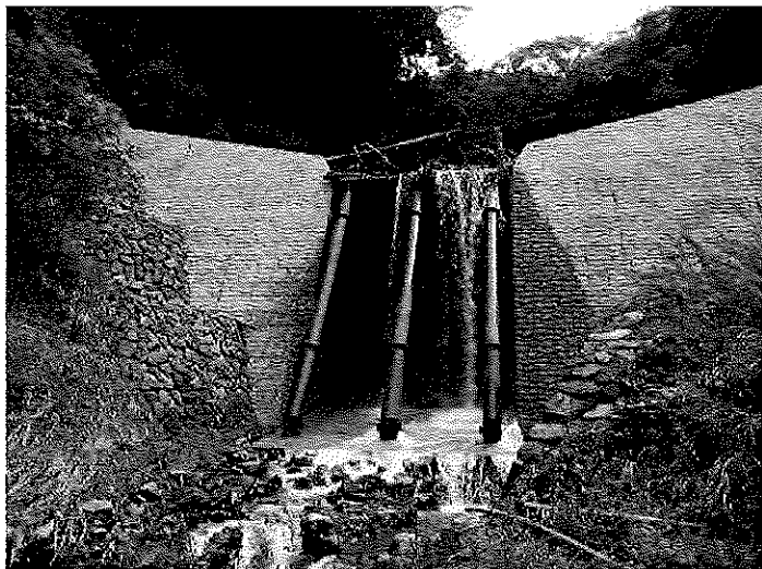
Examples of catching driftwood by open-type check dam
