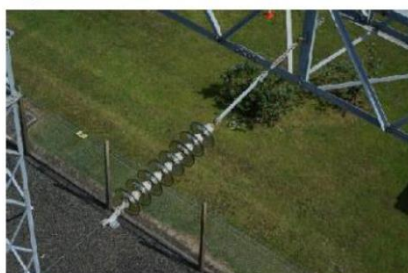
Top view of bus insulator
