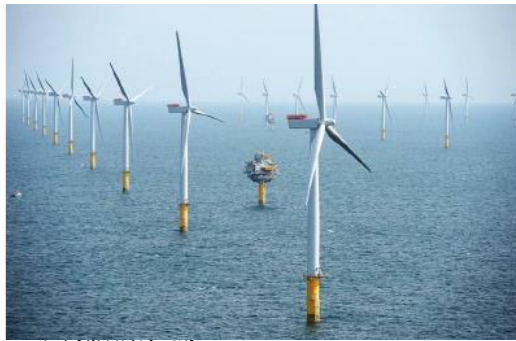
(風機間海纜 Inter Array Cable)
