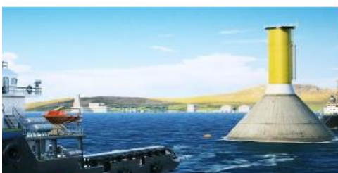
重力式結構(Gravity Base Structure)
