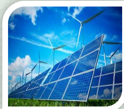
Production of Renewable Energy
