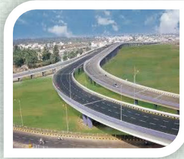
Construction of Road, Bridge and Railway Line
