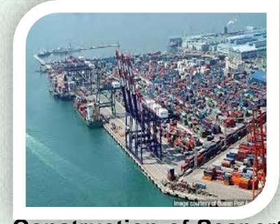
Construction of Seaport, River Port and Dry Port
