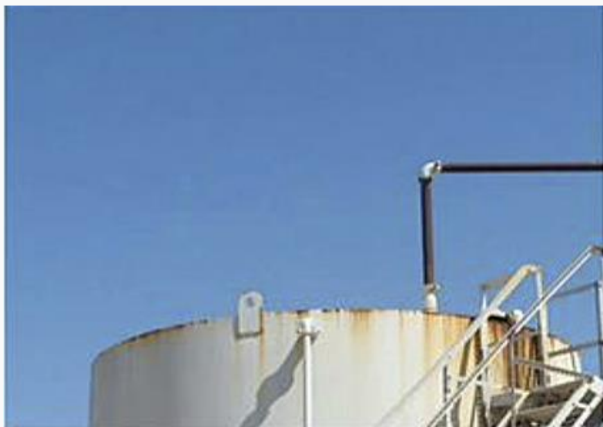
View of tank through naked eye.
