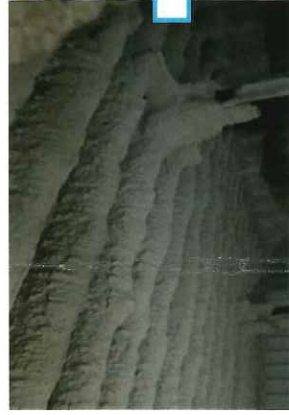
■ Cleaning with steam sootblower
