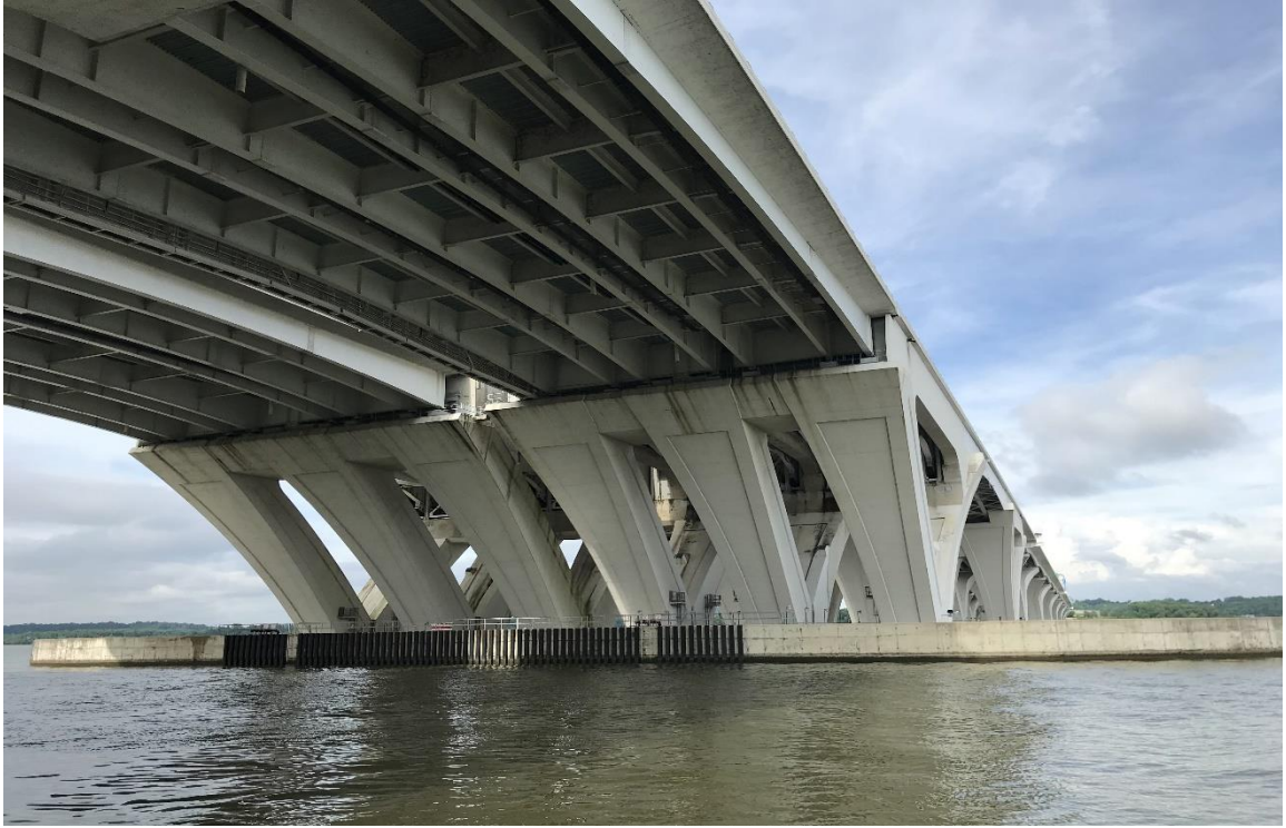
圖 3- 40 Woodrow Wilson Memorial Bridge
