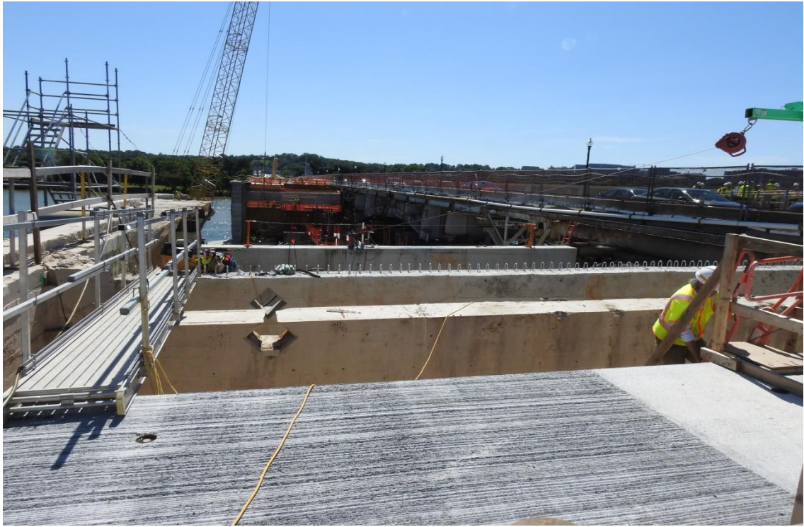
圖 3-32 Arlington Memorial Bridge 預鑄橋版掃紋
