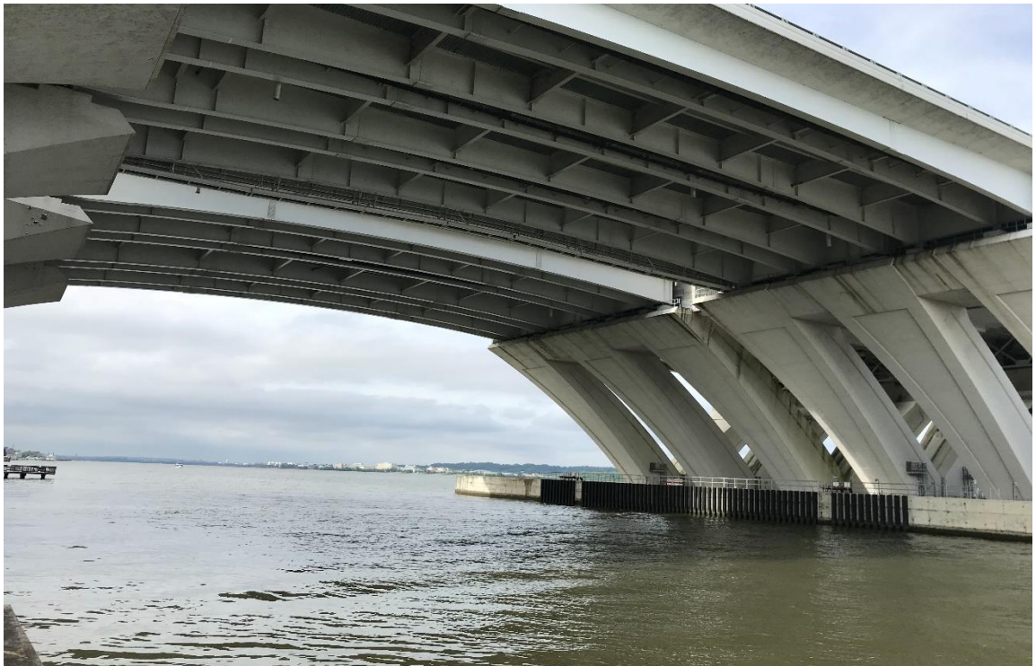
圖 3- 41 Woodrow Wilson Memorial Bridge
