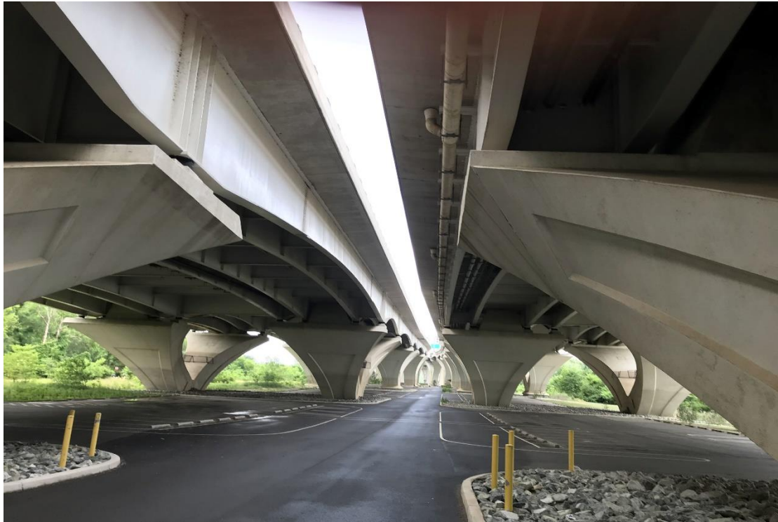
圖 3- 36 Woodrow Wilson Memorial Bridge
