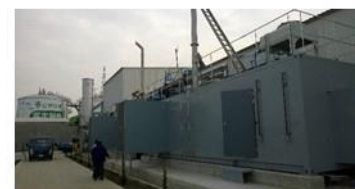
Kaohsiung, Chicken farm, biogas power, 400 kW e × 2 (feed-in grid)
