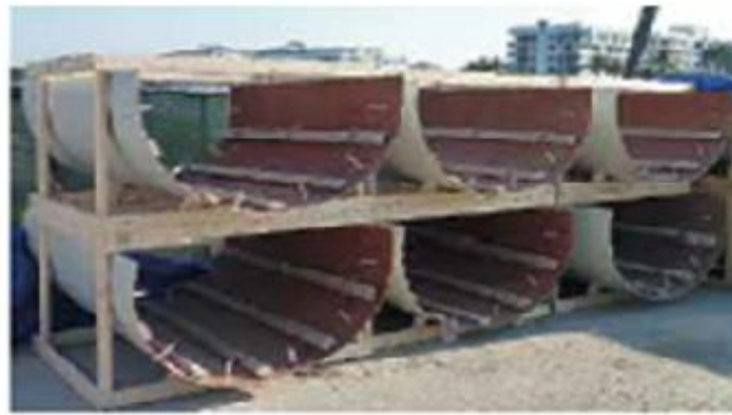
Galvashield DAS Jackets Prior to Installation
