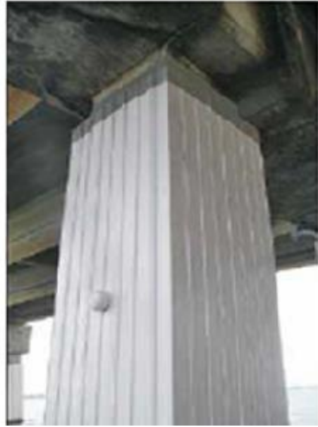
Tidal Plus Jacket with Modular PVC Stay-in-Place Formwork
