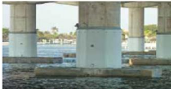
Galvanode DAS Jackets Installed
