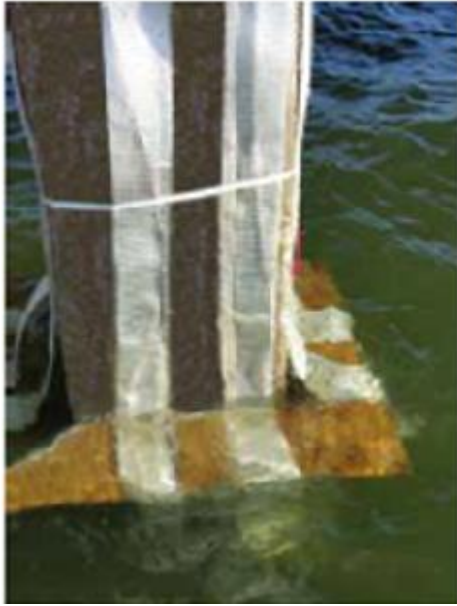
Tidal Plus Jacket with Wicking Fabric Anodes (prior to jacketing)
