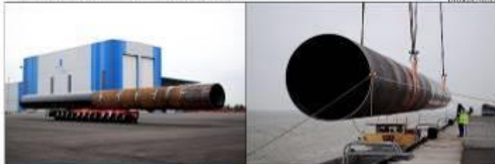
31 Pin Piles Ø 2.5m, length up to 50m, weight up to 100t
