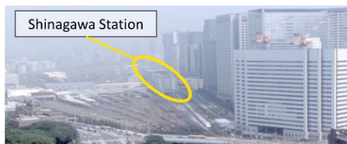
After opening of Shinagawa Station (2003)
