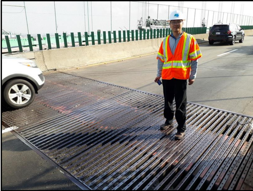
超大伸縮量的豎齒型伸縮縫(Vincent Thomas Bridge)
