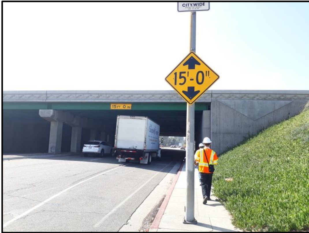
Western Ave Bridge
