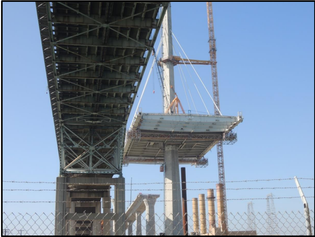
橋梁下方仰視 New Gerald Desmond Bridge 施工現況(左側為舊橋)
