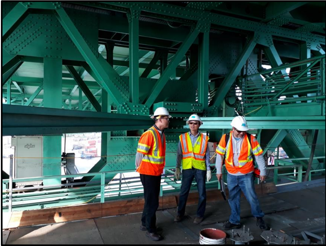
邊跨鋼橋油漆鋼橋更新作業(Vincent Thomas Bridge)
