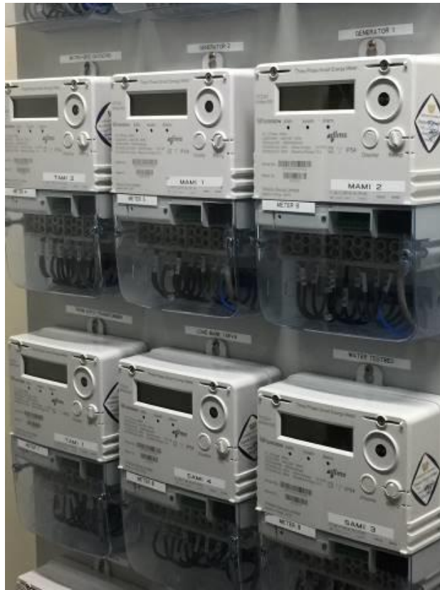
圖 5 : Electric Power Intelligent Control (EPIC)Testbed
