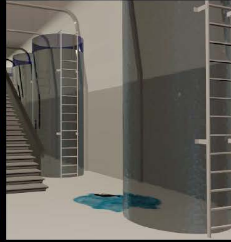
Water Leak in Aquaponic Unit 03
