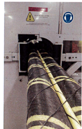
2 x HVDC + FO cables after bundling
