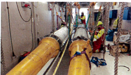
Simultaneous In-line jointing of 2 x HVDC cables
