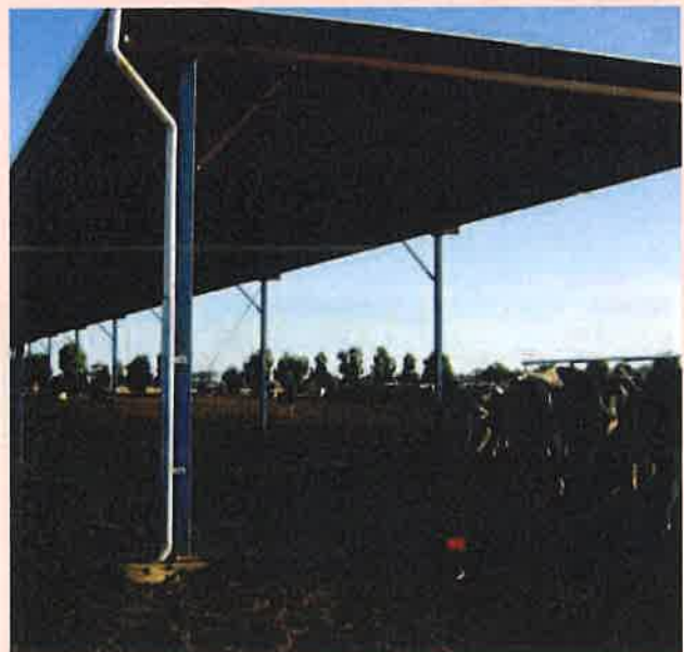
Water falling on the shade shed roof flows into gutters, then into several downpipes and underground piping that is directed to the recycle system. No stormwater from the roof lands on the feedpad floors.
