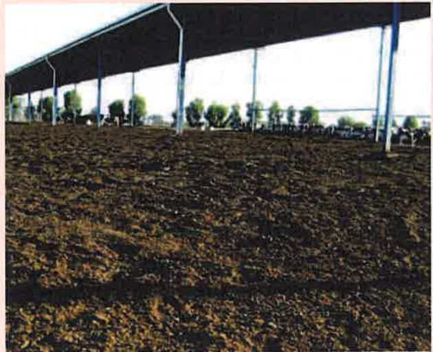
The ground slopes away from the drive alley and shade sheds at about 5-6% to enhance drainage.
