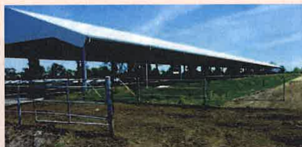
Permanent covered concrete feedpad with iron roof and a central, open ridge vent in the roof apex.
