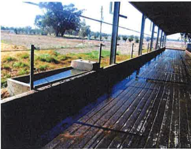
Note the position of the water trough, grooving to help prevent cow's slipping, water run-off from the roof to lane, high eaves and pitched roof to facilitate ventilation. The shed runs north-south to use sunlight to dry cow standing areas.
