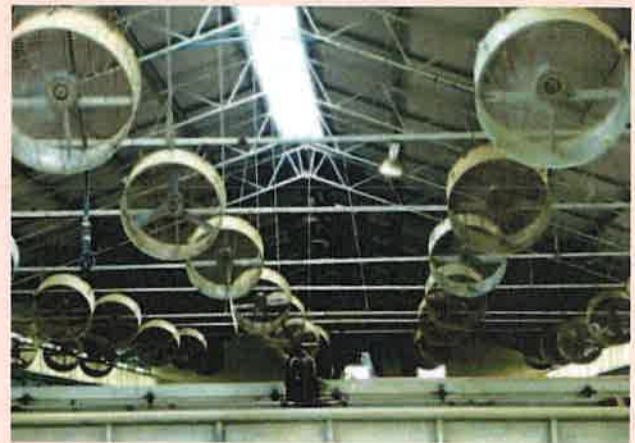
Fans set 2.3 m above cows, angled down. All fans push air from west to east with the prevailing wind.
