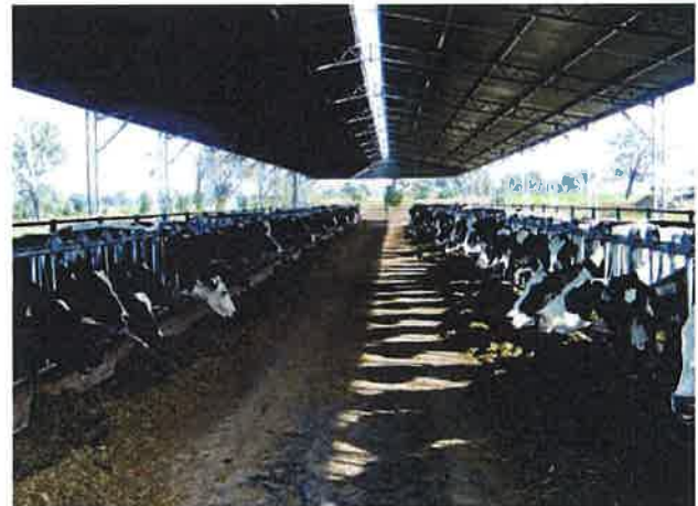
Sprinklers could be fitted above head lock stalls or at the back of the cow alley in the shed.
