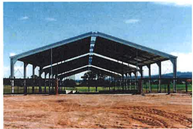
This roof slope is 18° with a 500 mm vent at the apex. Eaves are 4.3 m high, and 6.9 m at apex. The shed runs north-south with 3% slope on patterned cement floor. Feed troughs are 1.2 m wide inside, 400 mm high and 100 mm thick.
