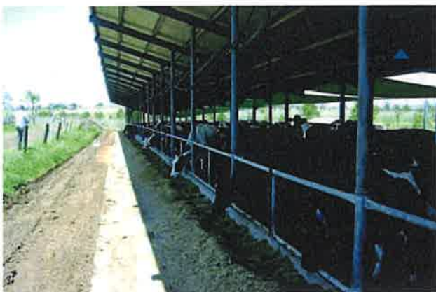
Note that the sprinklers above the feed line spray onto the cows' backs. The feedpad runs north-south and has a sloping roof to reduce the western sun projecting into the cow resting area.
