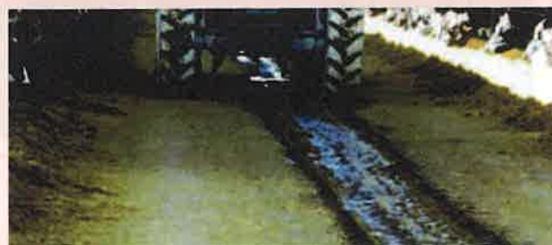
Central drive alley sloped to the centre to prevent rainfall that comes through the ridge vent contaminating the feed.
