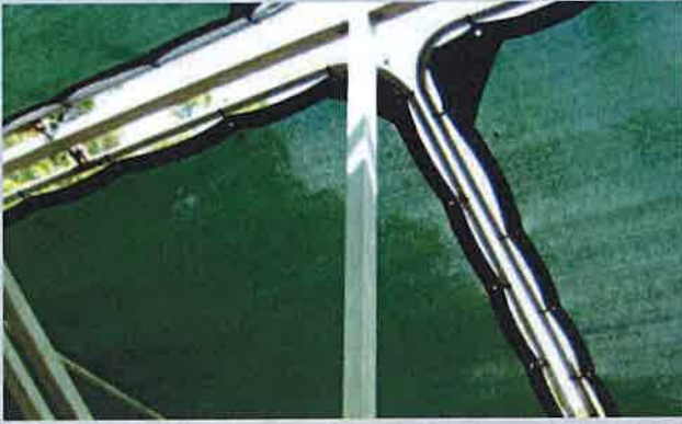
Hooks and eyelets attach the shade cloth securely to the frame. Struts ensure that flapping is kept to a minimum.
