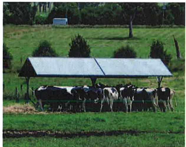
An iron-roofed structure will re-radiate heat on the cows underneath, so where possible create a larger gap between the cows and roof.
