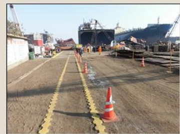
Secure evacuation routes with permanent marking
