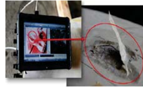
Surface damage detection of wind blade
