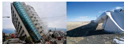
Building and Wind turbine collapse under earthquake (Source: windAction)
