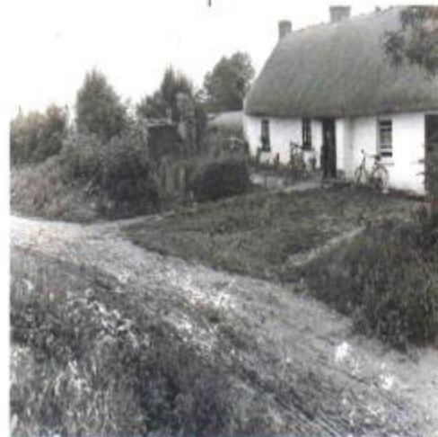
Rucky Hill (Dundalk to Carrickmacross Road) Road Improvement Scheme, 1938. Louth Local Authorities Archives Service
