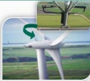
Wind turbine (Germany)
