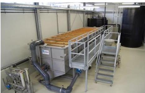
**EDAF** (Enhanced Dissolved Air Flotation) Remove SS up to **6000** mg/L
