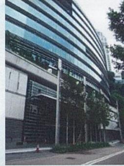
Hong Kong Electric Centre, Kennedy Road
