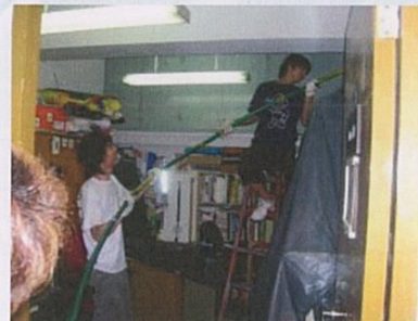
Duke of Windsor Social Service Building, Wan Chai
