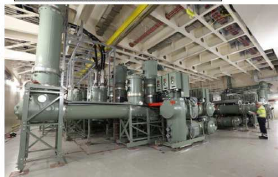
© 2017 General Electric Company. Proprietary. All Rights Reserved. 155 kV GIS Room
