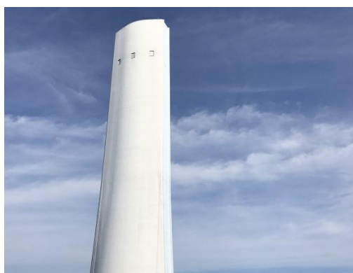
(a) J-POWER 磯子火力發電廠煙囪
