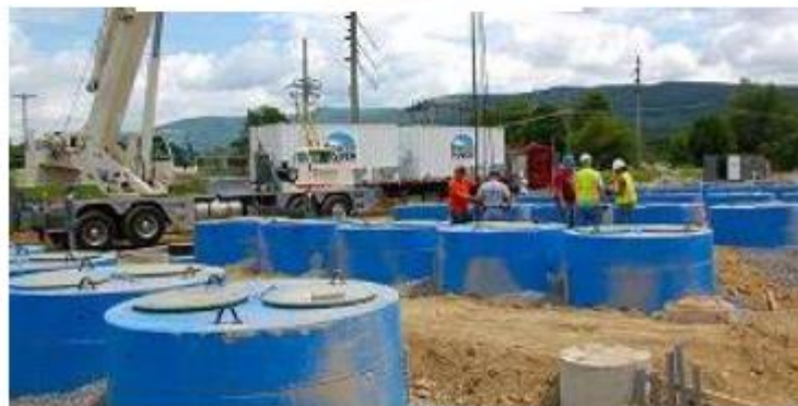
Construction of a Beacon plant
