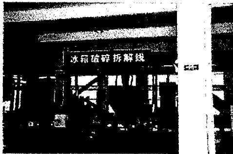
Refrigerator smashing and dismantling line
