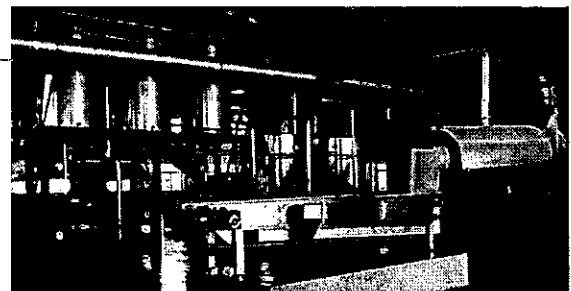
Test food waste treatment plant in Haiyan,
