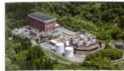
Yanaizu-Nishiyama Geothermal Power Plant (Photo courtesy of Tohoku Electric Power Co., Inc.)
