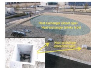
FREA Ground-Source Heat Pump System Demonstration Area
