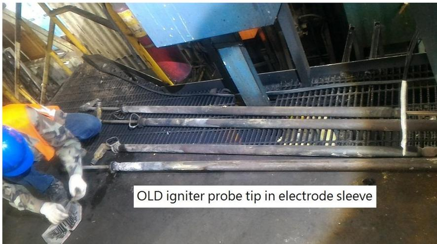
FIGURE 11. OLD IGNITER PROBE TIP IN ELECTRODE SLEEVE
