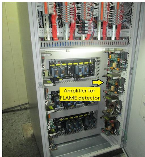
FIGURE 30.AMPLIFIER FOR FALEM DETECTOR
