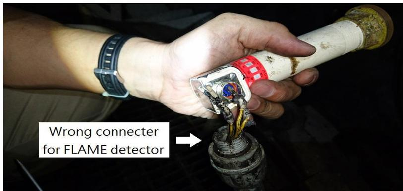
FIGURE 29.WRONG CABLE CONNECTER FOR FALEM DETECTOR
