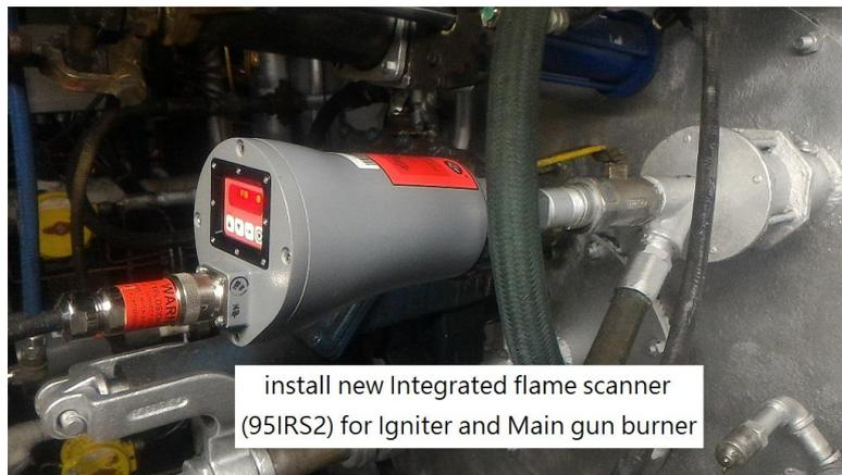
FIGURE 30.AMPLIFIER FOR FALEM DETECTOR
