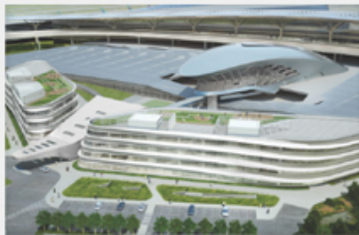
2 The 2nd Administration Building
