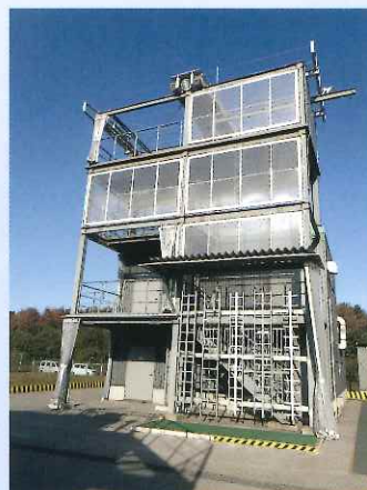
A: 風車安全教育設備 Work at Height Training Facility
