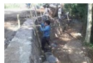
Retaining Walls 38.184 Unit
