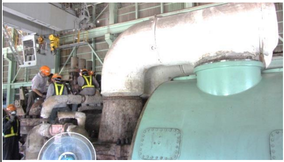
HP inlet pipe assembly
