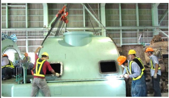
HP inlet pipe assembly
